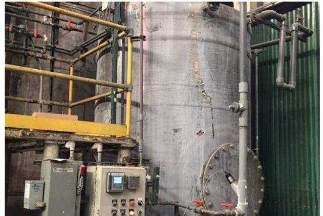
If the scrubber uses strong caustic (10-15% NaOH), pH control is not suggested since the exposure of the pH glass to high concentration of caustic will attack the pH glass, thus destroying the electrode. The pH response curve follows a strong acid/base titration curve, which results in a reading that only drops back on-scale near a point of complete exhaustion of the caustic, followed by a sudden drop at the exhaustion point.
